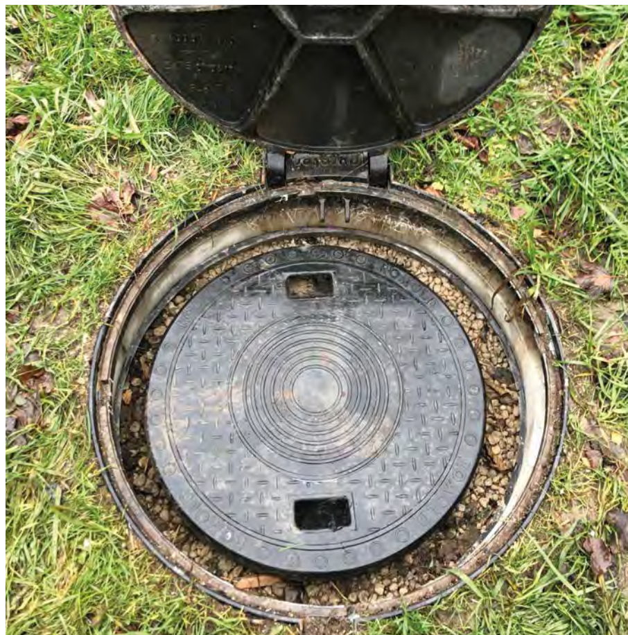
Das ROMOLD Deckel-in-Deckel-System
